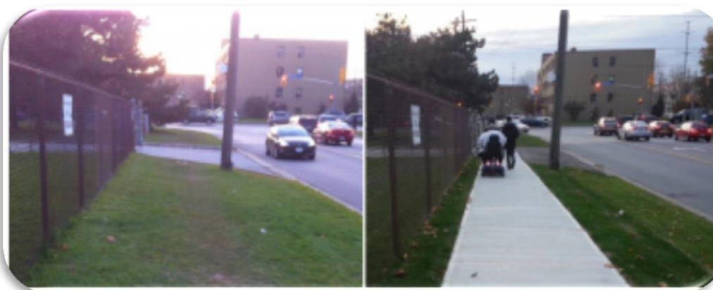
Missing Links Sidewalks
