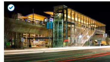
Transparency and high quality lighting connects interior and exterior spaces, Aberdeen Station, Richmond.
