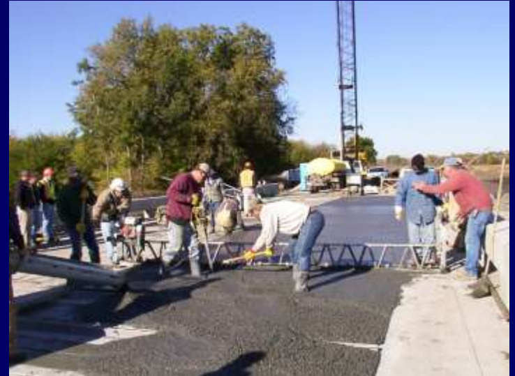
Conductive Concrete Slab
