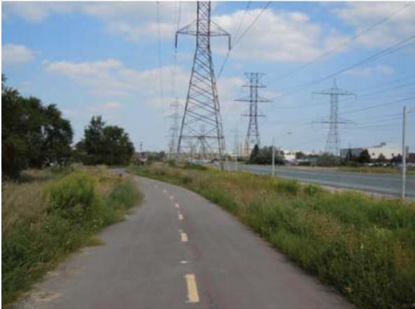
Figure 4: Sample Active Transportation Pathway / Multi-use Trail in Place of a Sidewalk on Roadway with Infrequent Crossings / Driveways.<sup>177</sup>
